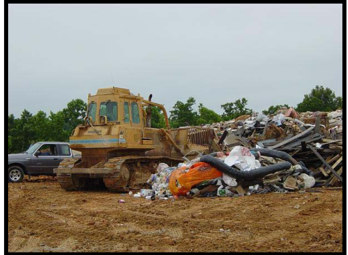
Municipal Solid Waste landfill in North Carolina
