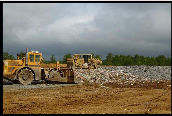
Municipal Solid Waste landfill in North Carolina
