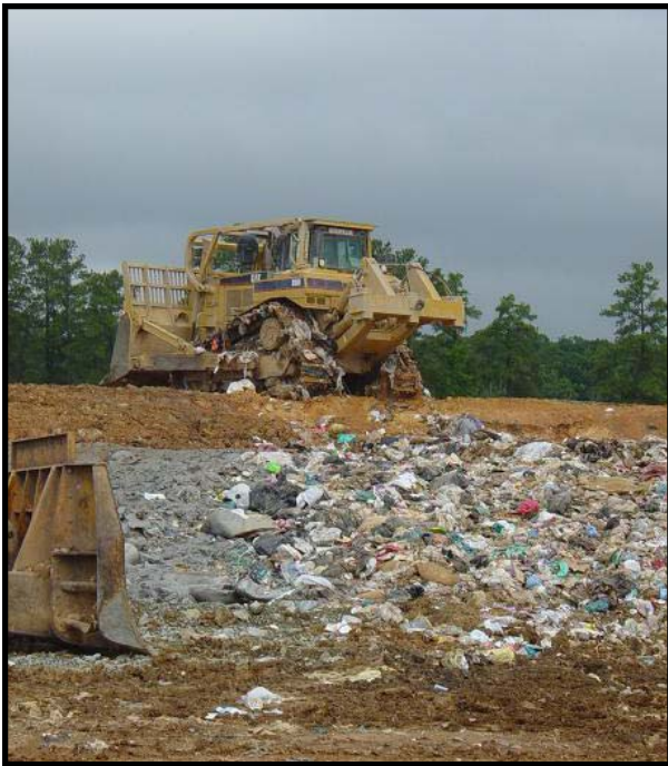
Compacting trash at a Municipal Solid Waste Landfill in North Carolina
